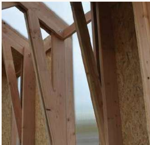
CHARPENTE — ASSEMBLAGES BOIS
