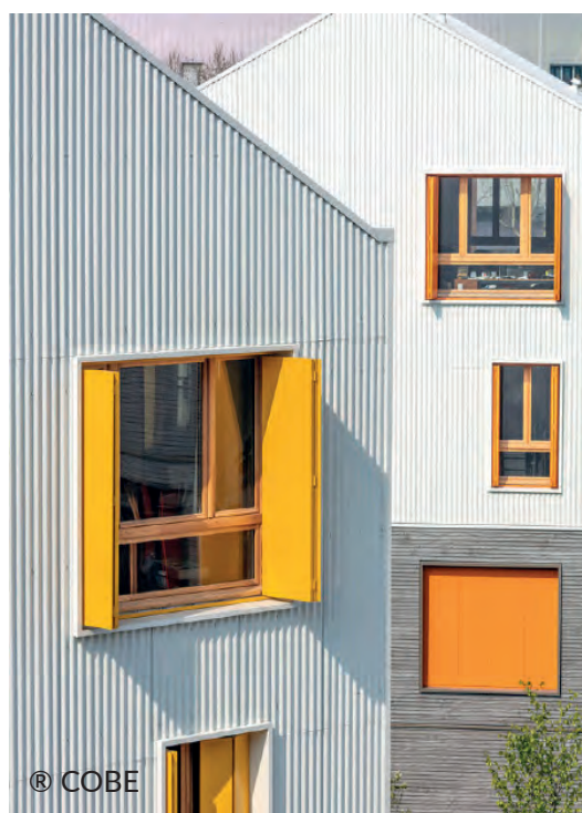
High-quality timber window frames enhance the building's material palette.
