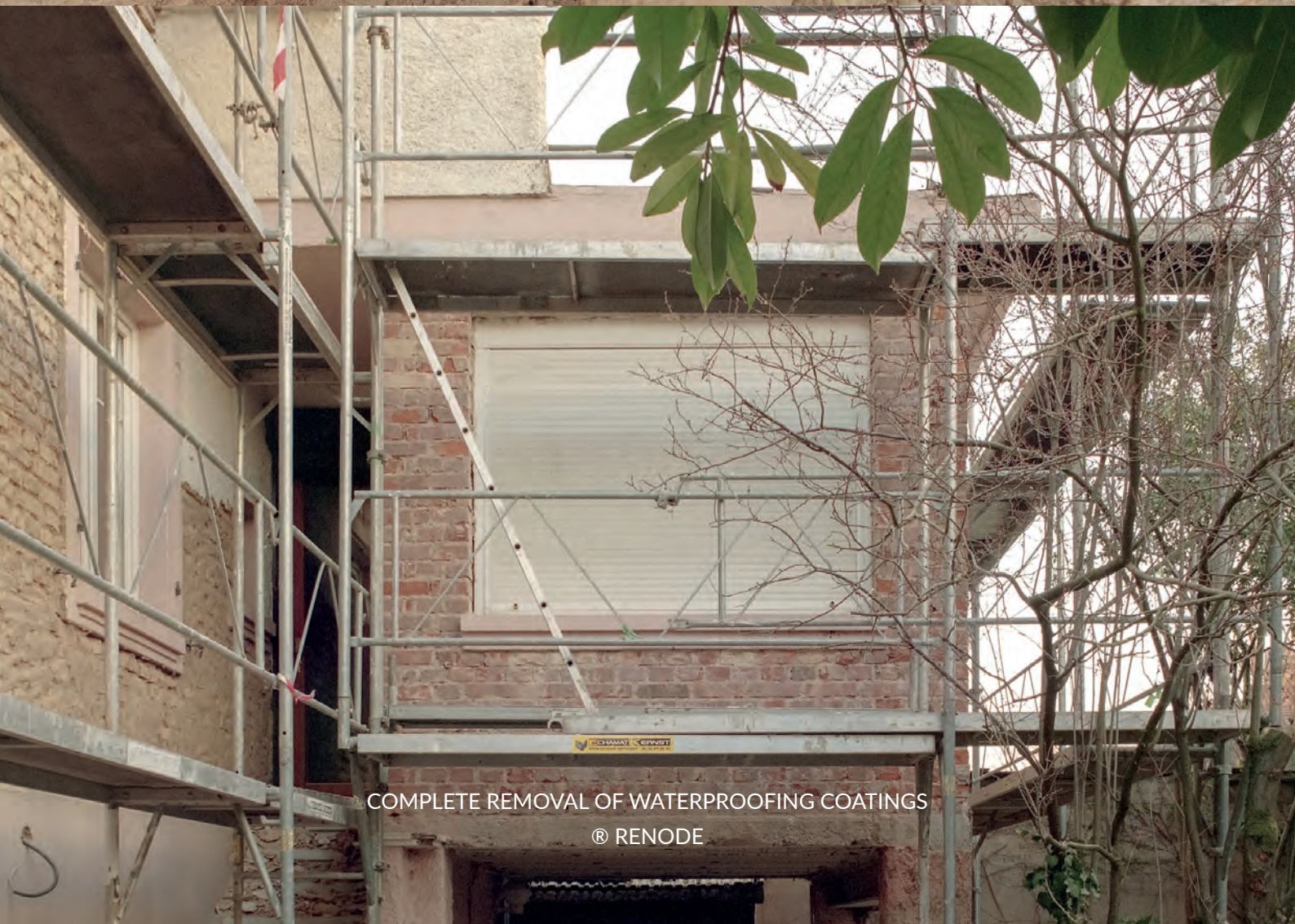
COMPLETE REMOVAL OF WATERPROOFING COATINGS ® RENODE
