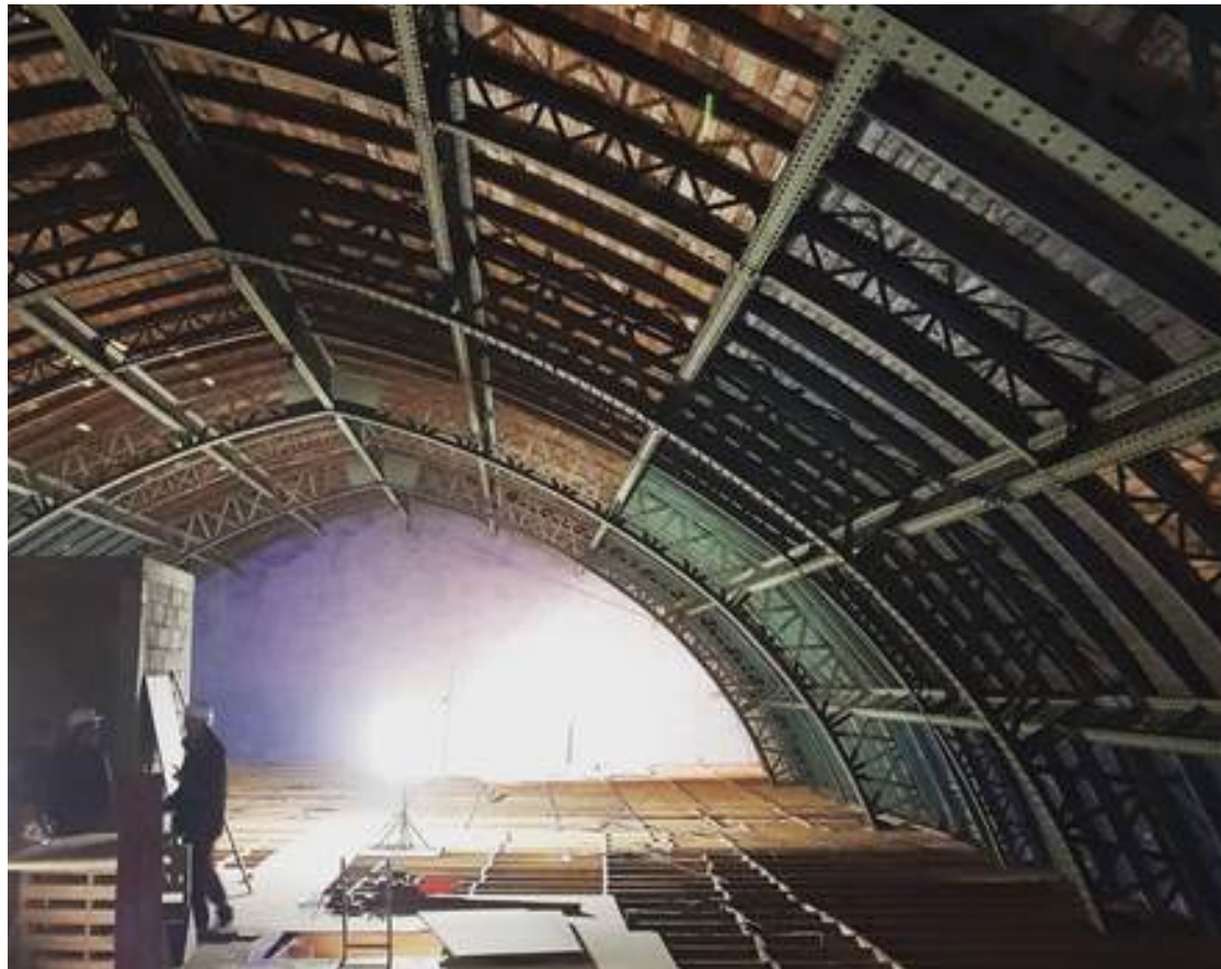
Structure Gustave Eiffel
