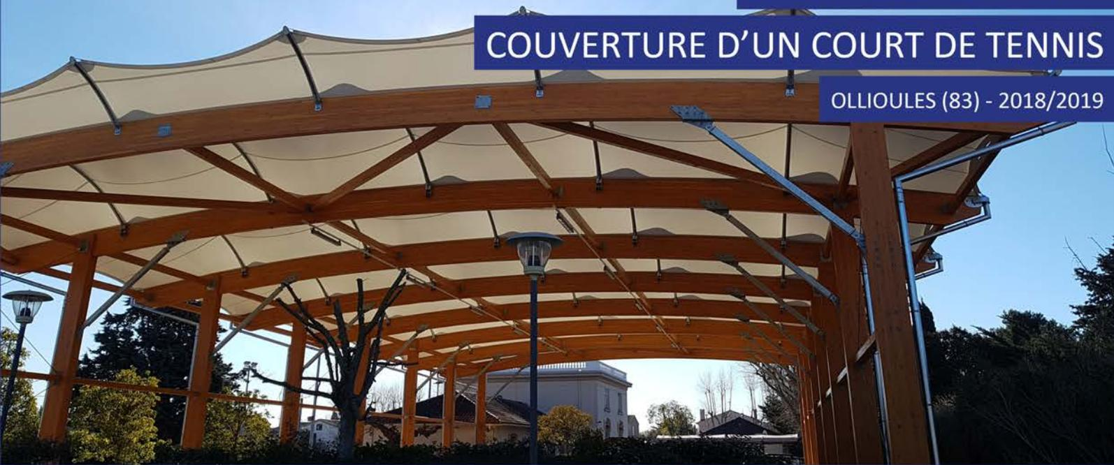
STRUCTURE PORTIQUES BOIS LAMELLÉ COLLÉ. COUVERTURE MEMBRANE TEXTILE TRANSLUCIDE A DOUBLE COURBE INVERSE.
