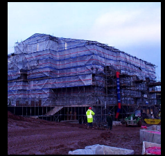
Construction Capricious Welsh weather dictated a fully protected construction
